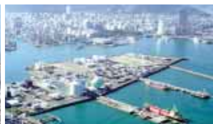
Takamatsu Plant, Shikoku Gas.
