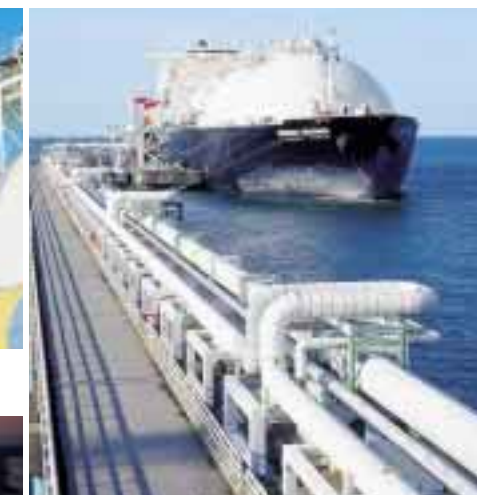
The Energy Advance berthing at the pier. A thick pipe connected to onshore tanks is installed along the pier.
