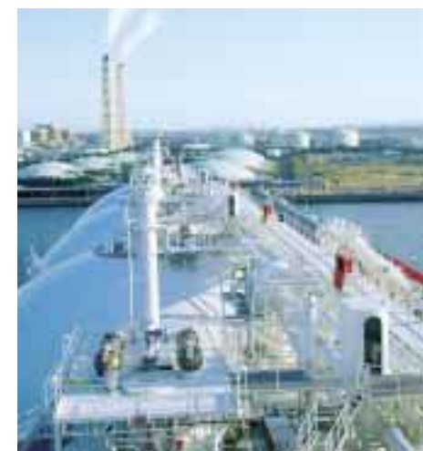
Sodegaura LNG Terminal seen from the bridge of the Energy Advance .
